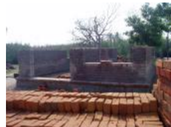
A house under construction with four-rod pillars
